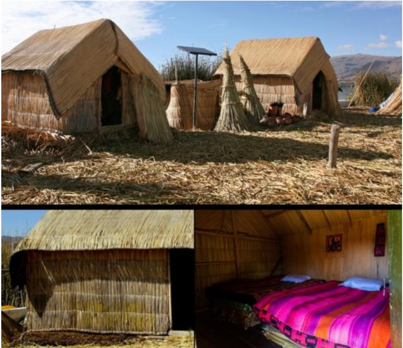
A home in the indigenous pre-Incan community in South America (the Uru or Uros people) made with woven-fiber technology.
