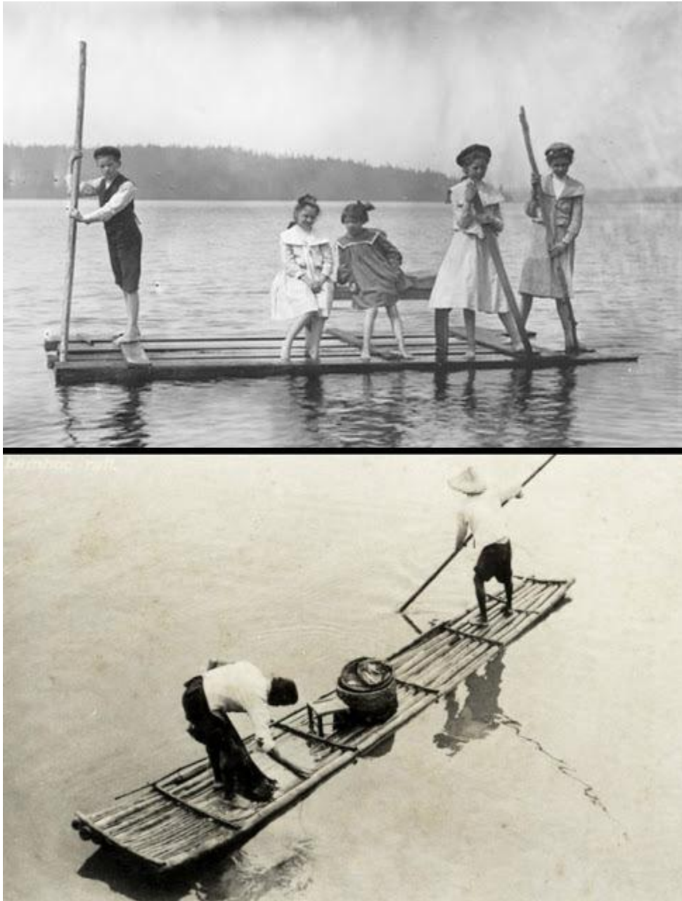
(Top) Children on a raft -- the crossbeams are clearly visible and keep the raft together. (Bottom) A common working bamboo raft in Taiwan. The horizontal right-angled slats are visible.
