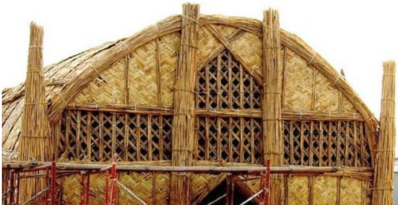
Detail of the front of a mudhif community building under construction.
