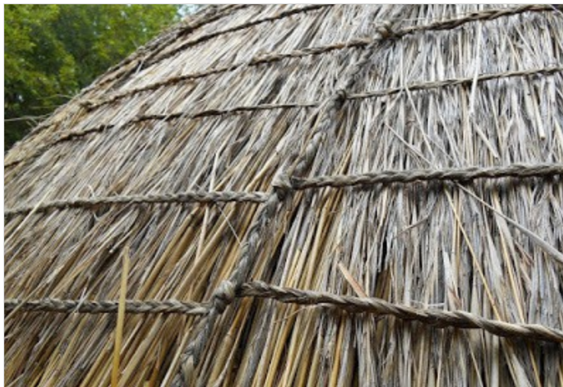
Detail of thatching of the replica Zulu hut (full view of Zulu hut is above bottom left).
