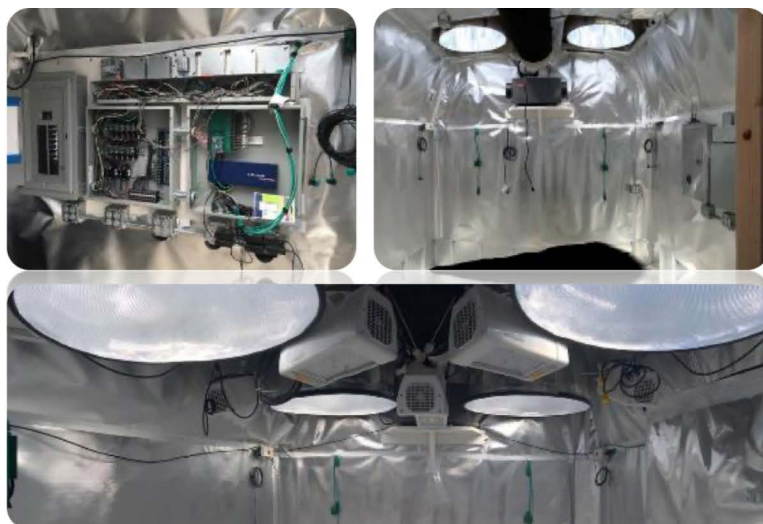
Figure 3 - Grow Room Intelligence - Control Panel & Circuit Breaker (top left), Climate Sensors placed around grow room (top right), placement of LEDs among SkyVaults (bottom). Note, in top right photo Solatube SkyVaults are partially installed, without dimmer, amplifier or prismatic diffusers components.
