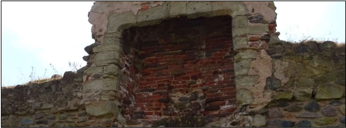
Figure 5.12 A brick fireplace at Grace Dieu built by John Beaumont. The missing fireback has exposed the original stonework. Photograph taken by author.
