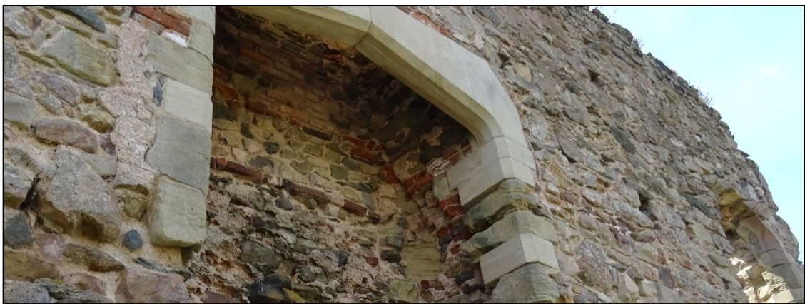
Figure 5.13 Another fireplace at Grace Dieu which has undergone modern conservation. The priory stonework is again exposed by the missing Tudor brickwork. Photograph taken by author.
