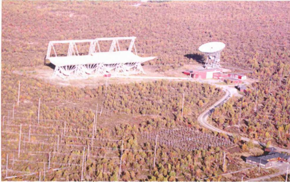
**Figure 4.1.** The EISCAT site at Tromsø, Northern Norway. The UHF transmitting antenna is in the top right of the picture and the VHF is in the top left. The heater array is in the bottom left of the picture.
