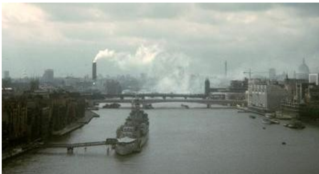
Figure 5.4: ‘Plume droop’ at Bankside, c.1973.
