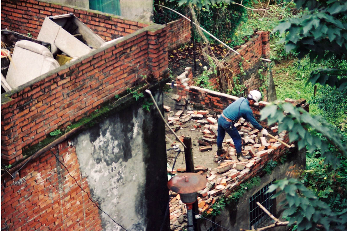
Figure 4.7 The partial demolition in April 2002. In order to prevent associated collapses of other self-constructed buildings from partial demolition, the City Government agreed to tear down some houses by hand. Photo taken by the author in 2002.
