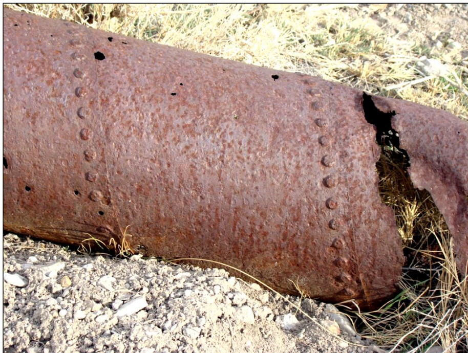
Figure 3-21. Remnant of 21-inch Spiral Riveted Pipeline at the Wah Wah Reservoir
