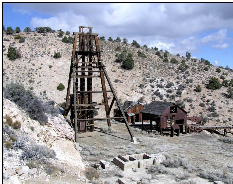
Figure 2-24. Headframe, King David Mine, Frisco, Utah (Photograph by Author, June 2009)
