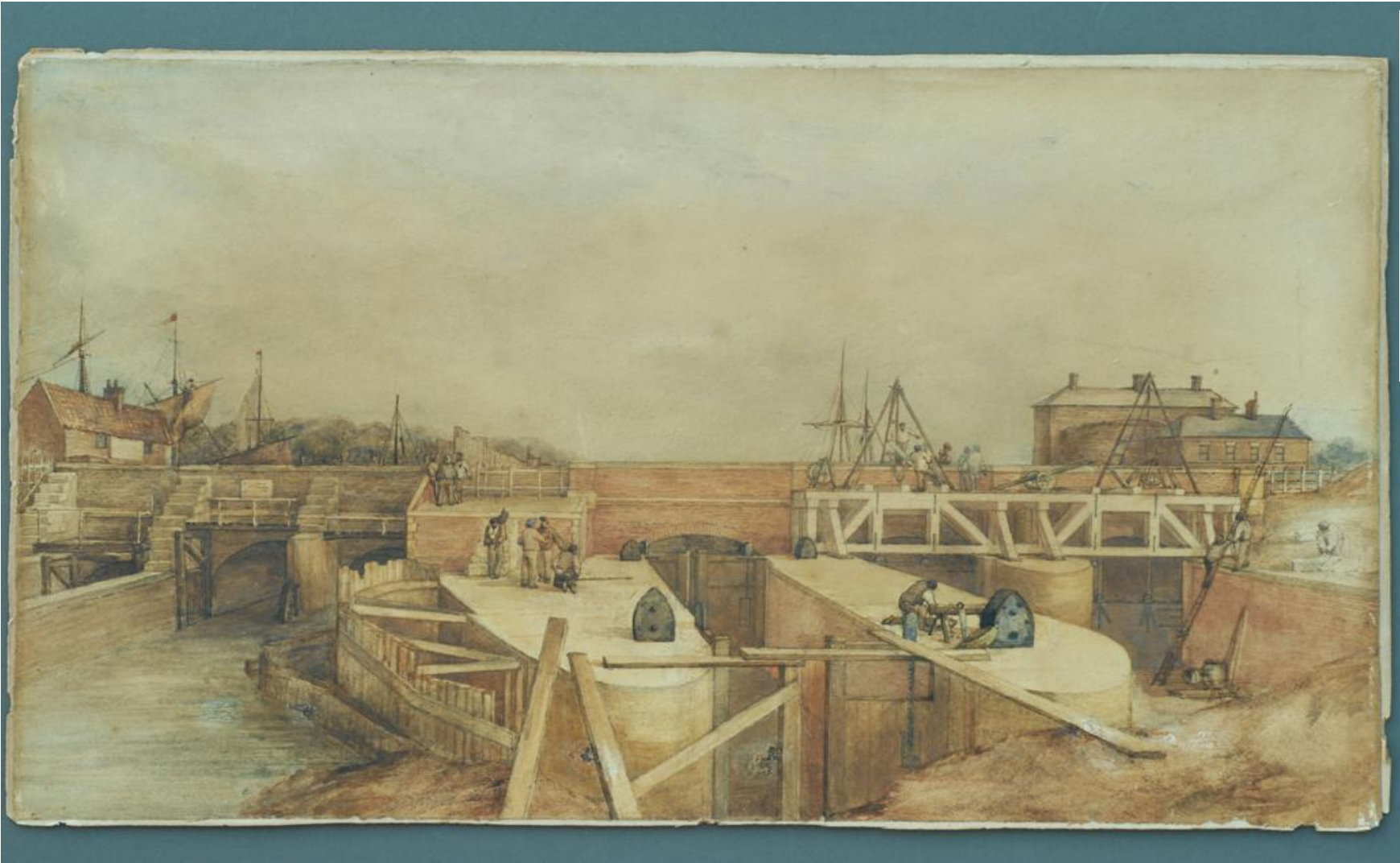
William Lewin painting of the third Black Sluice (centre and right) under construction 1847-8. On the left is the second Black Sluice, built 1765 upon the site of the 17 th century sluice. William Lewin (1794-1863), a surveyor and civil engineer, was also resident engineer to the River Witham Commissioners. My thanks to Lorraine Heyes for this copy of the painting.
