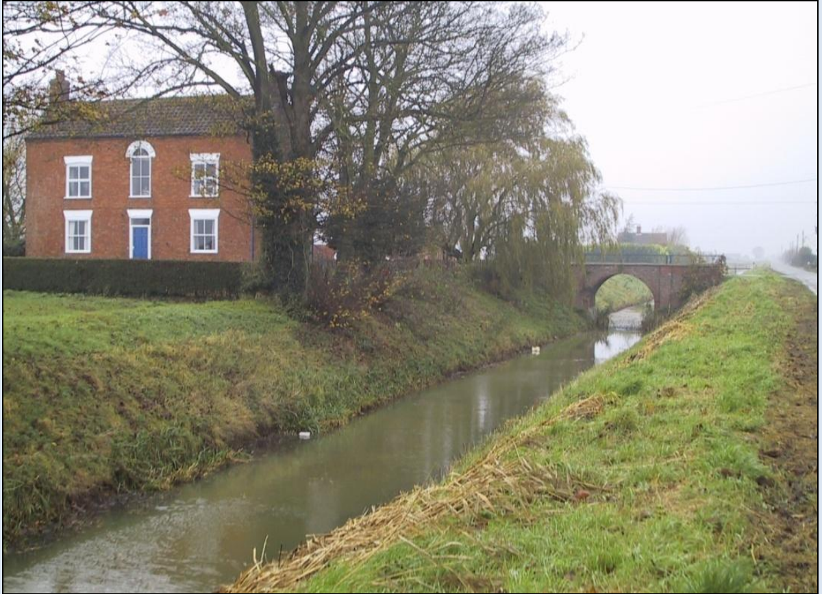
Figure 3.10. One of the original bridges over the North Forty Foot drain. The high arch allowed small packet and carrier boats to pass underneath. Kirton Fen is on the left with the North Forty Foot Bank road from Toft Tunnel to Chapel Hill, just visible on the right.
