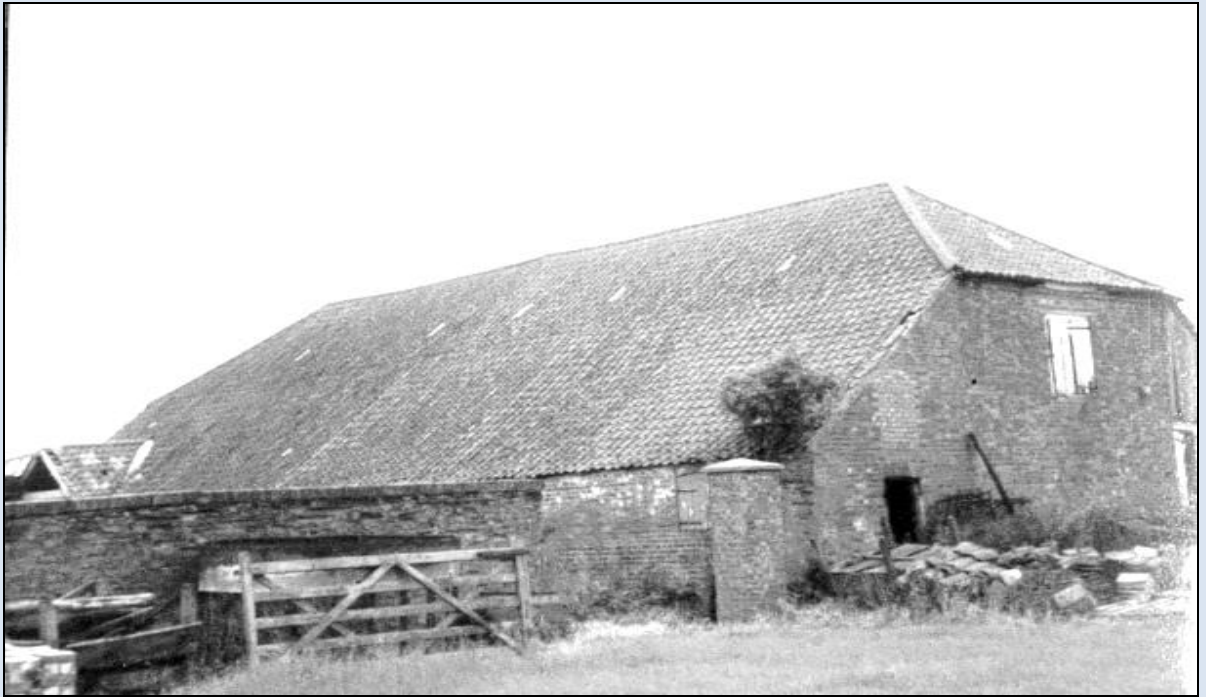
Figure 3.9 Catslider roof on the northern side of the crew-yard, Terry Booth Farm
