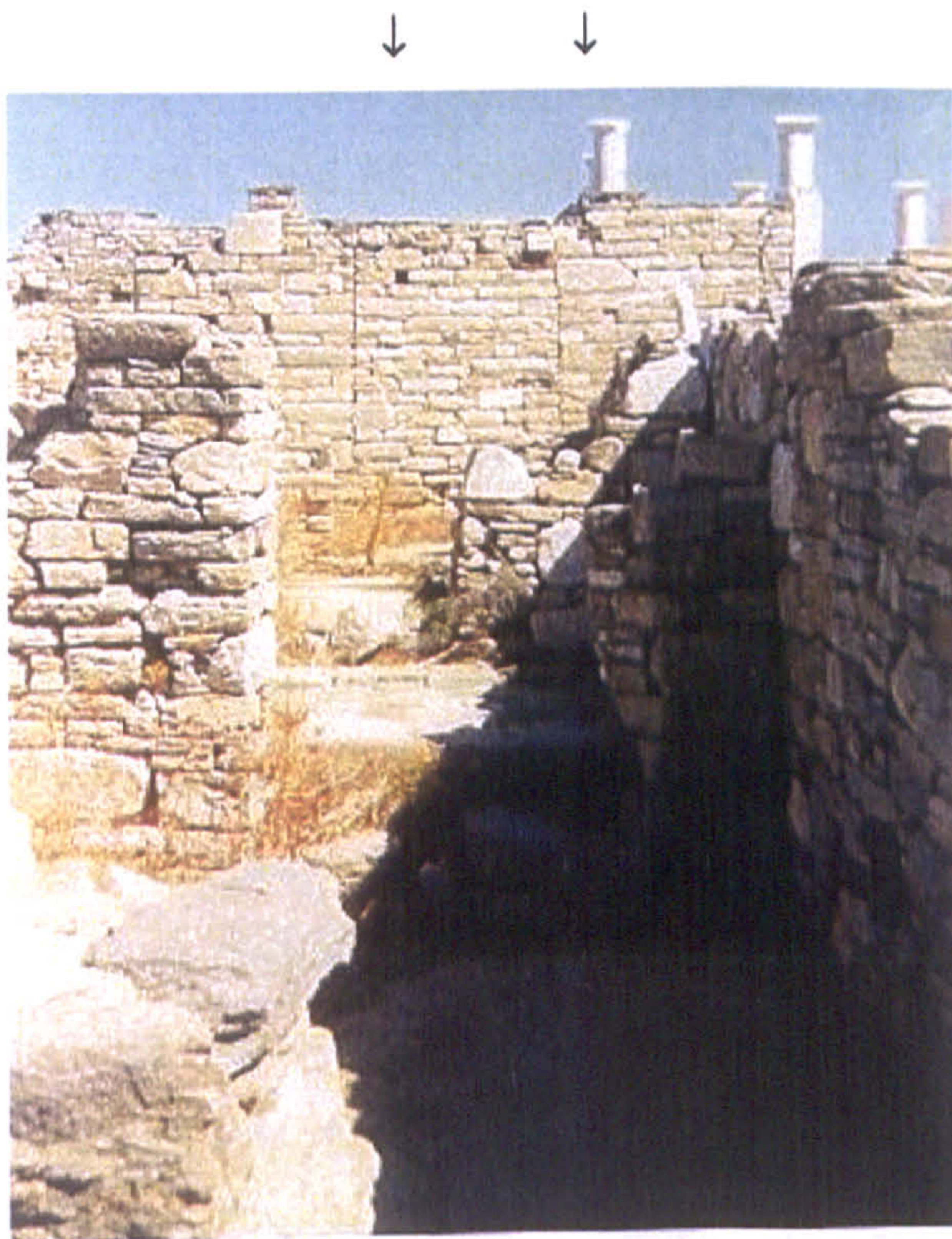
Figure 64: Blocked doorway opening in VI d's exterior wall, viewed from within Insula III. The arrows indicate the edges of the blocked door.
