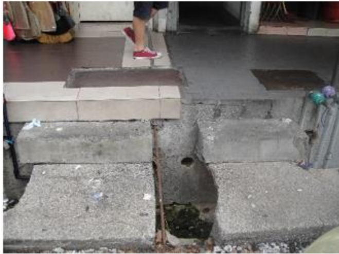
Figure 4.11: Damaged and uneven steps bridging a drainage between the road and walkway along several eateries. (Location: Damansara Jaya)
