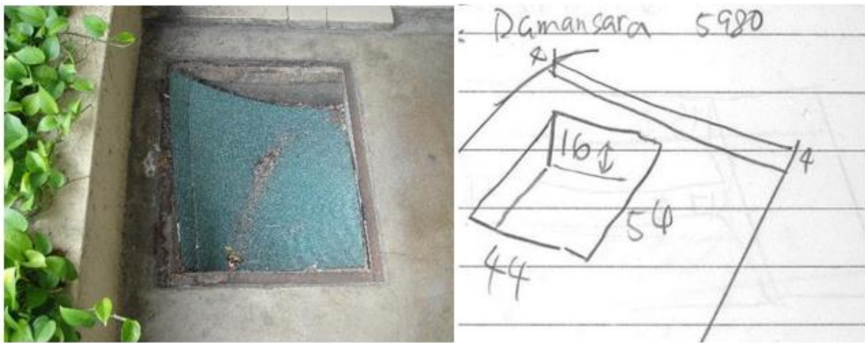
Figure 4.10: A pit along a walkway connecting several private services, uncovered and hazardous. (Location: Kota Damansara)
