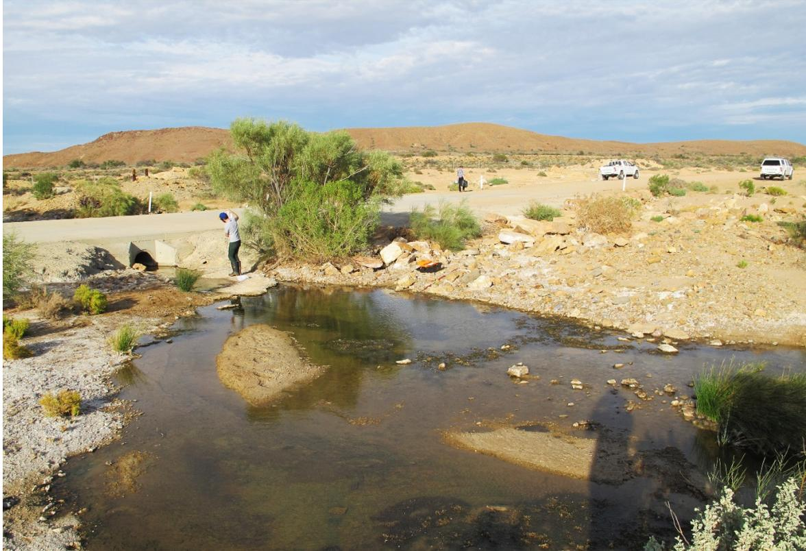
**Figure 12.** A pool formed as a result of a raised roadway in the Lake Eyre Basin, in which several fish species were found. While a culvert is present, it was disconnected from the main pool.
