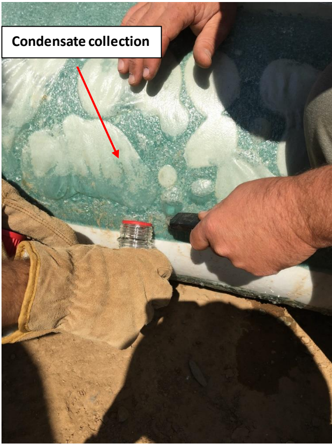
Figure SI-8. Water diffused through the thickness of the CIPP liner during CIPP installation
