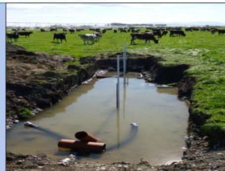
**3. Plumbing** - Install pipes and connect bioreactor to inflow, outflow and overflow structures, as required.
