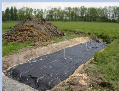
**5. Bioreactor cover** - Depending on soil type and other local conditions, a geotextile cover should be installed, especially if farming will continue over bioreactor. Top the bioreactor with soil.
