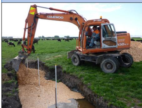
**4. Woodchip addition** - Digger fills in bioreactor with wood chips.
