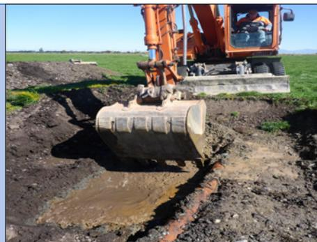
**2. Site preparation** - Earthworks to dig the bioreactor pit. Lining the bioreactor with geotextile fabric depends on the heaviness of soils.
