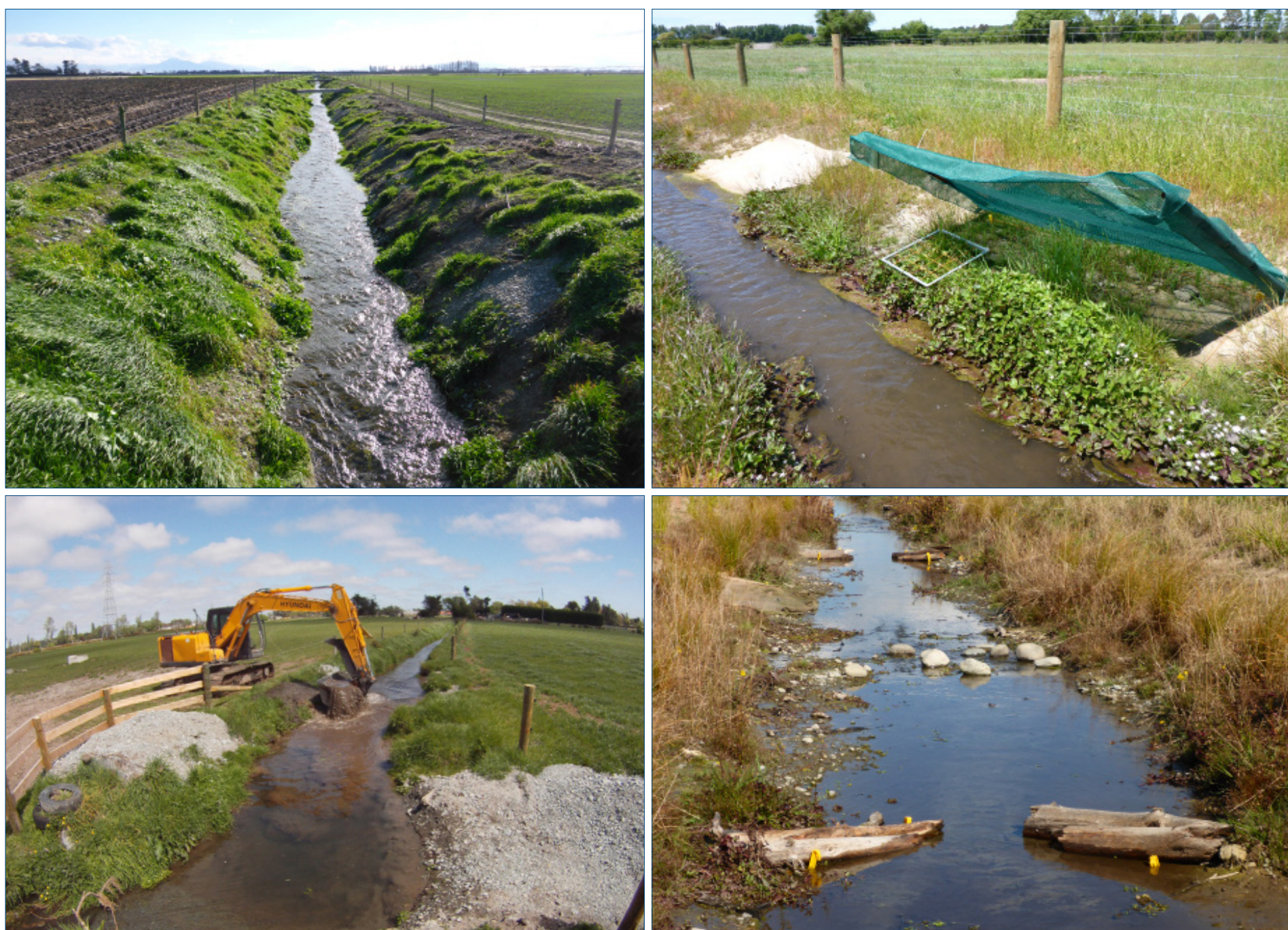
Trials include macrophyte control experiments, constructing sediment traps, and addition of in-stream habitat.
