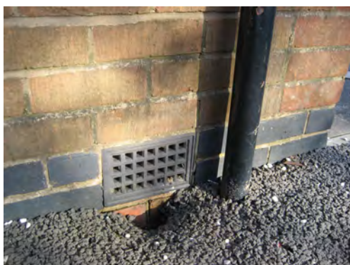
(a) Sub-floor air brick photograph.
