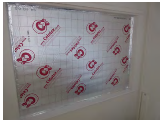
(d) Insulation blocking east and west facing windows. Sealed with aluminium tape.
