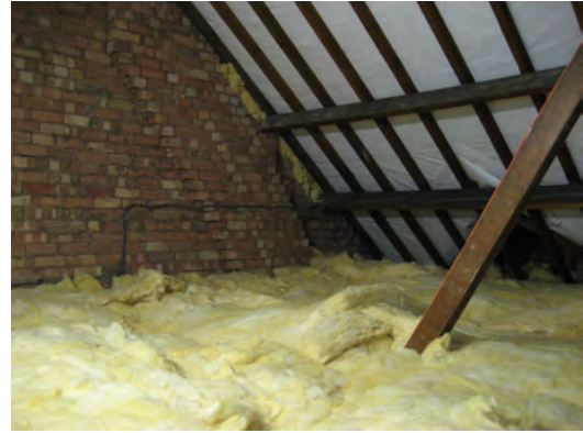
(b) Internal view of loft space. Glass mineral wool insulation at joist level and vapour membrane at rafters. Party wall visible to rear of photograph.
