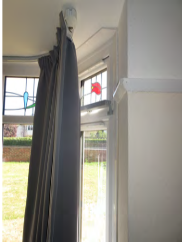
(a) Gap between living room curtain and wall as observed with curtains closed.
