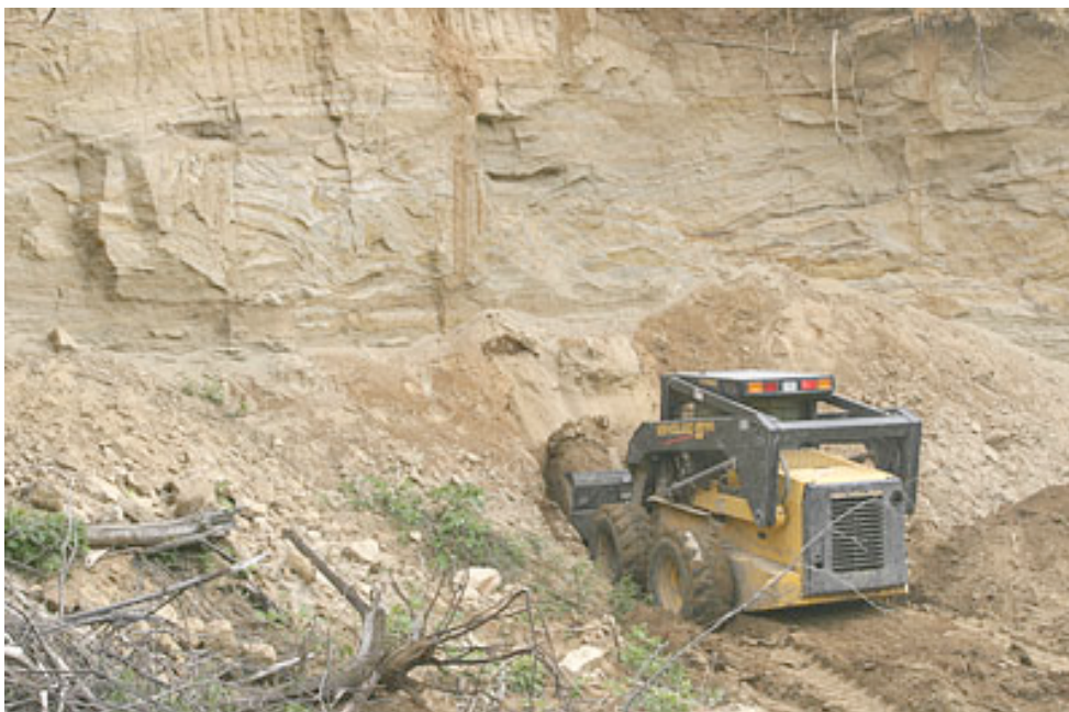
Figure 3.3C. Landowner using front-end loader to remove the lower 2 m of cover at Kulas Quarry.
