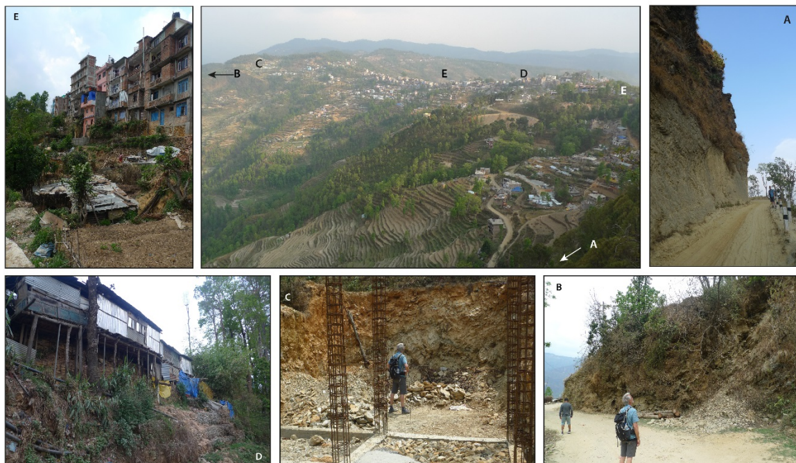
Figure 9. Central image provides a context for the ridge-top urbanised community of Chautara. (A) Vulnerable and exposed access road beneath a steep rock wall to the north of the town. (B) An active landslide at the southern edge of the town. Local people reported that the large block moves every monsoon and impacts the road. (C) Conditions for excavating foundations are challenging. The surface material comprises weathered and fractured bedrock, and has been affected by slope movement. (D) Informal housing at a slope edge, illustrating the challenges of building where flat space is limited. (E) There is a lack of flat building space at the town edge and buildings are constructed several storeys high at the slope edge. British Geological Survey (c) UKRI 2020.
