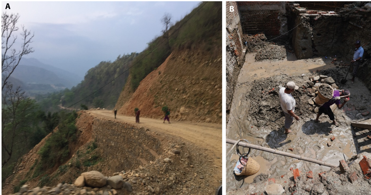
Figure 7. (A) The road that accesses communities on the Salyantar terrace is cut into a steep escarpment that is vulnerable to instability during monsoon rains. (B) Excavation in silts and fine sands with a sump pump, for building foundations in Bhaktapur in April 2018. Evidence for liquefaction below the feet of the construction workers. Local people reported that this stage of reconstruction is not possible during the monsoon.
