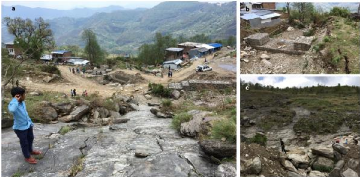
Figure 8. The community of Phulkarka is at risk from high stream flow, overland flow and landsliding. (A) The slopes above the community are widely stripped of their soil cover and this results in very rapid and destructive floods during the monsoon. A system of gabions is being constructed to direct flows and reduce their erosion potential. (B) A close-up of a gabion structure intended to control flow in a stream channel. Bank stability is still very poor (large cracks are visible) and housing is in very close proximity to the stream channel. (C) an view of the slopes above the community highlights the absence of suitable slope and vegetation cover. It is reported that the treeline visible to the left were planted by the community in an attempt to stabilise a landslide.
