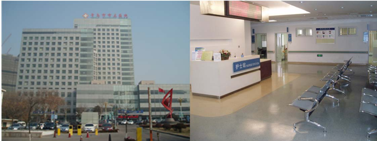
Figure 1: Interior and exterior views of one of the surveyed hospitals.
